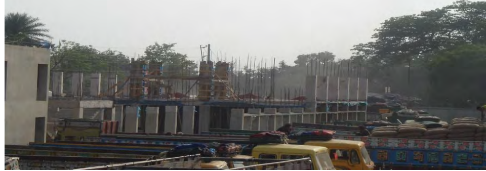
Administrative Building under construction
