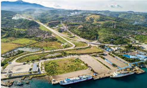
Strengthening Infrastructure to Support Economic Development and Basic Services
