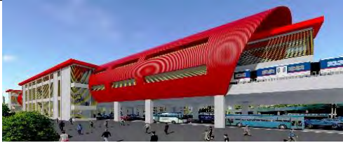
01 North Avenue (Elevated)
