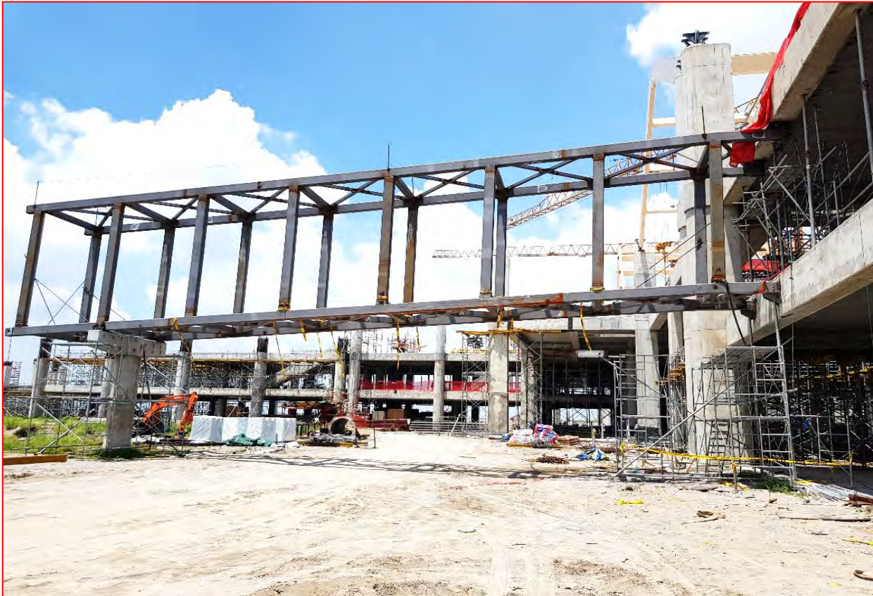
Figure 17: Fabrication and installation of Fixed Link Bridge (FLB – 13) in Building 4.
