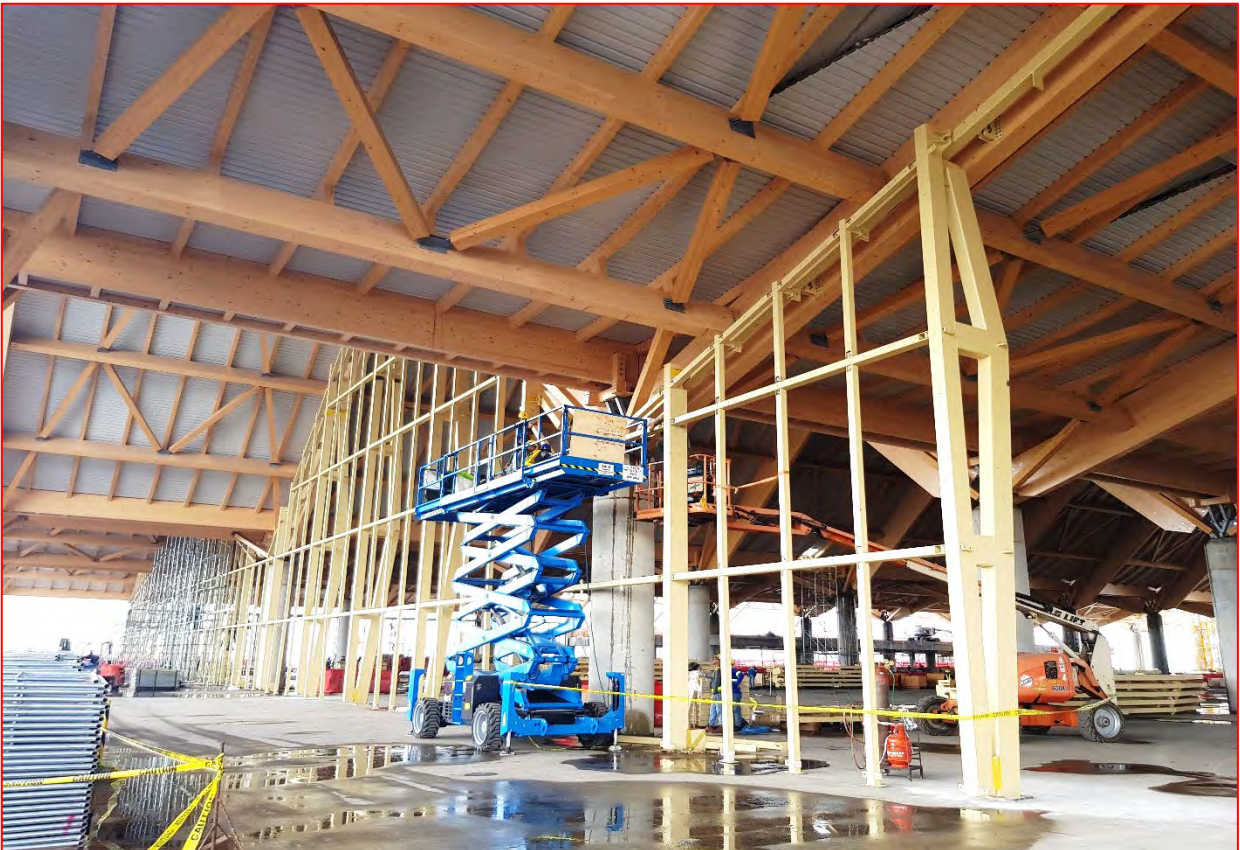
Figure 14: Façade Steel installation in GL 42 in Building 1 – West Pier.
