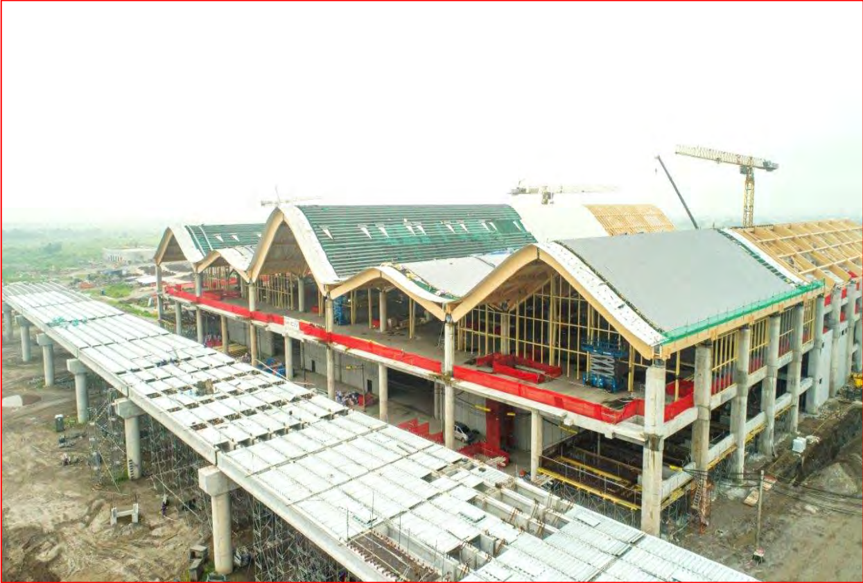
Figure 3: Roof Sheeting Final Layer – Riverclack installation in Building 1(a) – West Pier.
