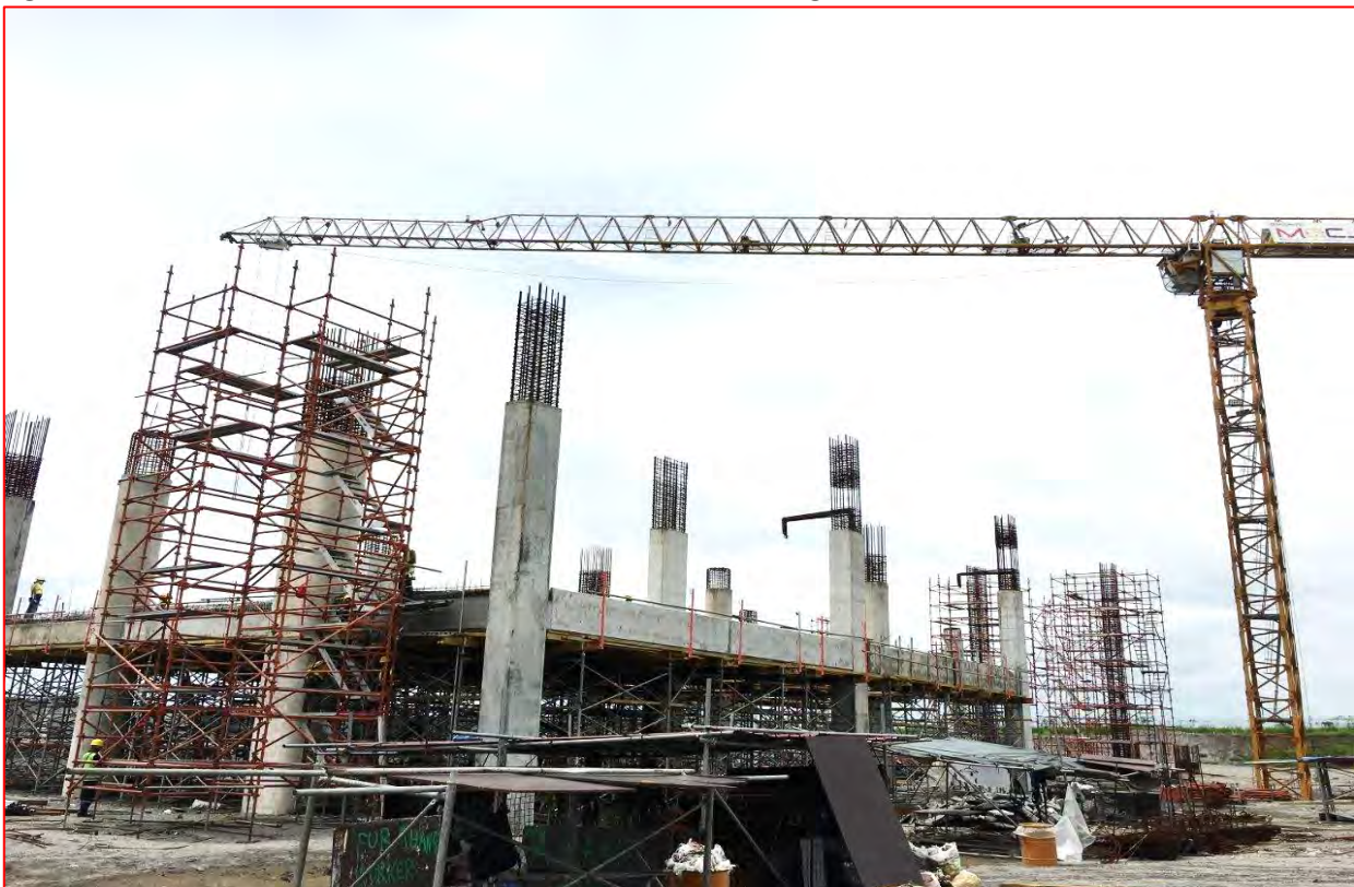
Figure 16: Arrival Level Beams and Slab construction in Building 3C – South Pier.
