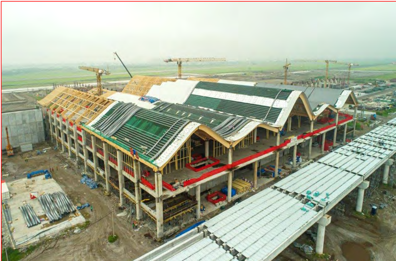
Figure 2: Building 1 – West Pier Roof Structure installation substantially completed.
