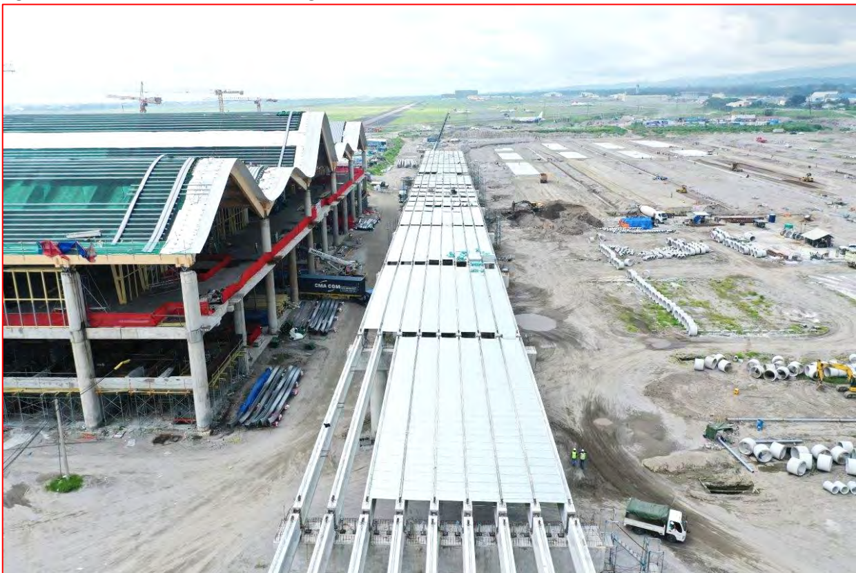
Figure 18: Elevated Road steel decking installation and corbel construction.
