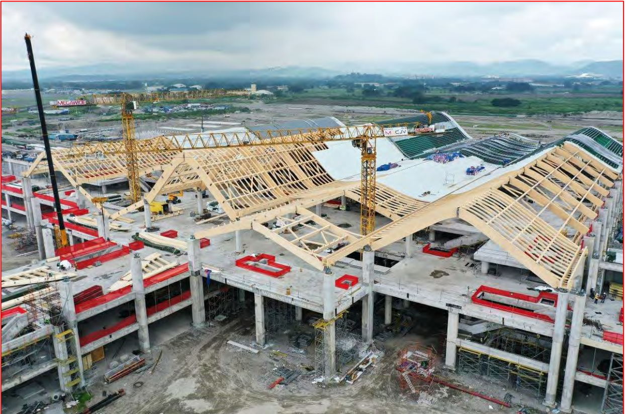
Figure 4: Departure Level concrete placing substantially completed in Building 1.
