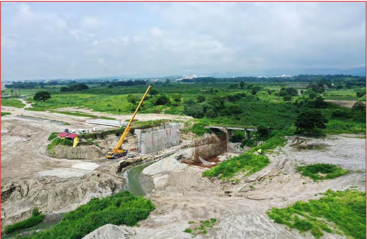
Figure 24: Civil/ Structural Substructure Construction of Dolores Bridge
