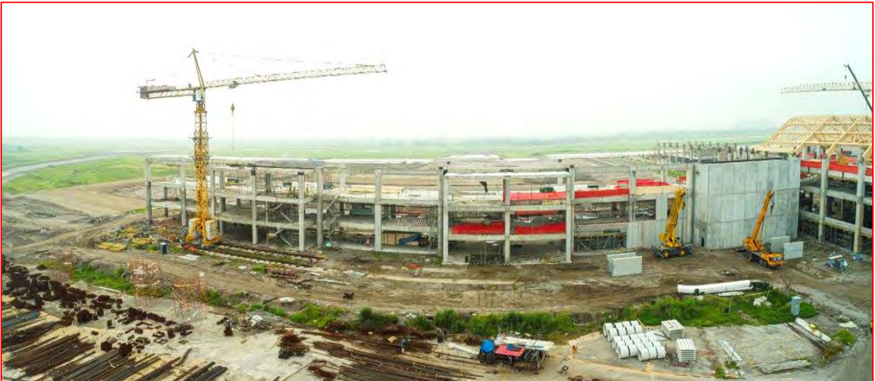
Figure 11: PC Wall Panel(Perimeter) and CMU installation in Building 4 – North Pier.
