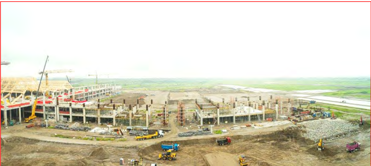
Figure 8: High/Roof column construction in Building 2 – East Pier.
