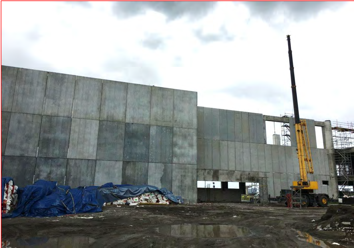
Figure 15: Precast Concrete Wall Panel installation in GL L-N along GL 31 & 32 in Building 3.
