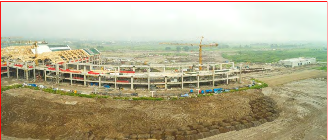
Figure 12: Structural Completion on Arrival/Departure/Roof Level in B4 – North Pier Building.
