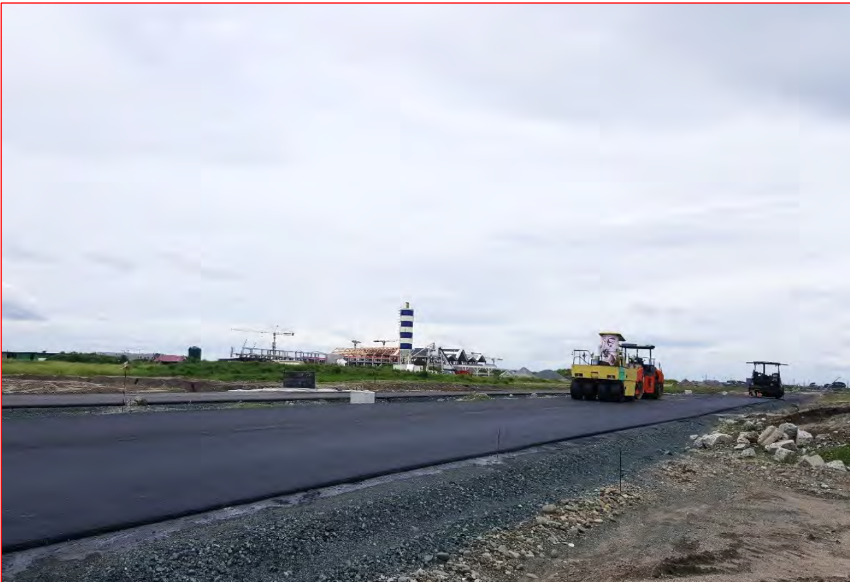
Figure 22: Asphalt laying and compaction in Main Access Road.
