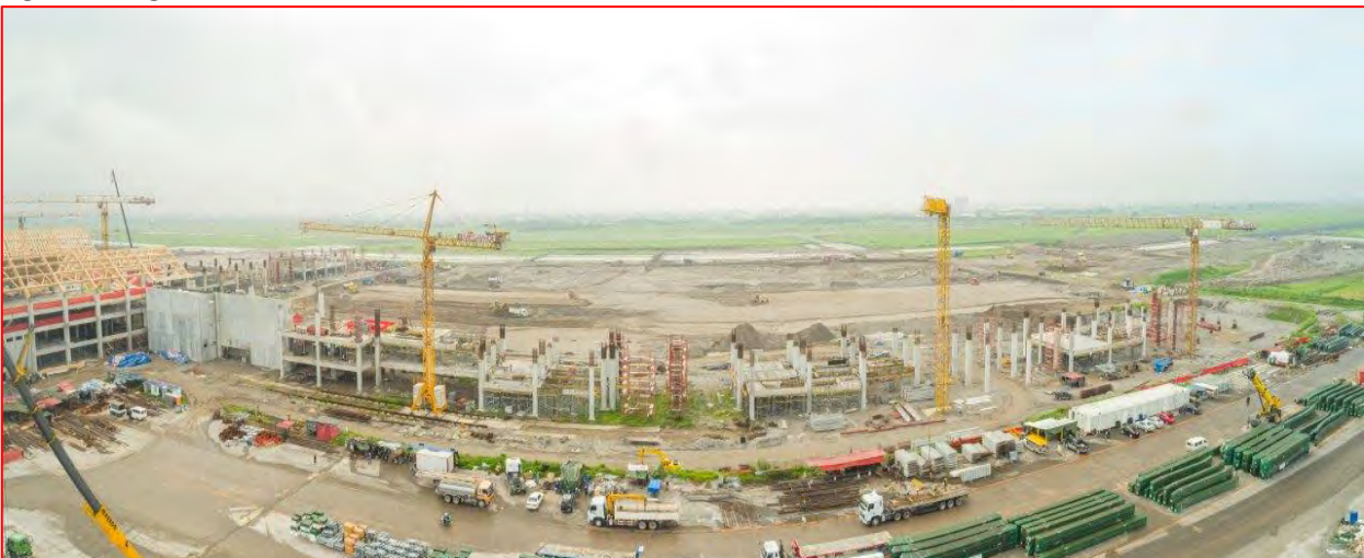
Figure 9: High Column/Beams/Slab construction and PC Wall Panel(Perimeter) installation in B3– South.
