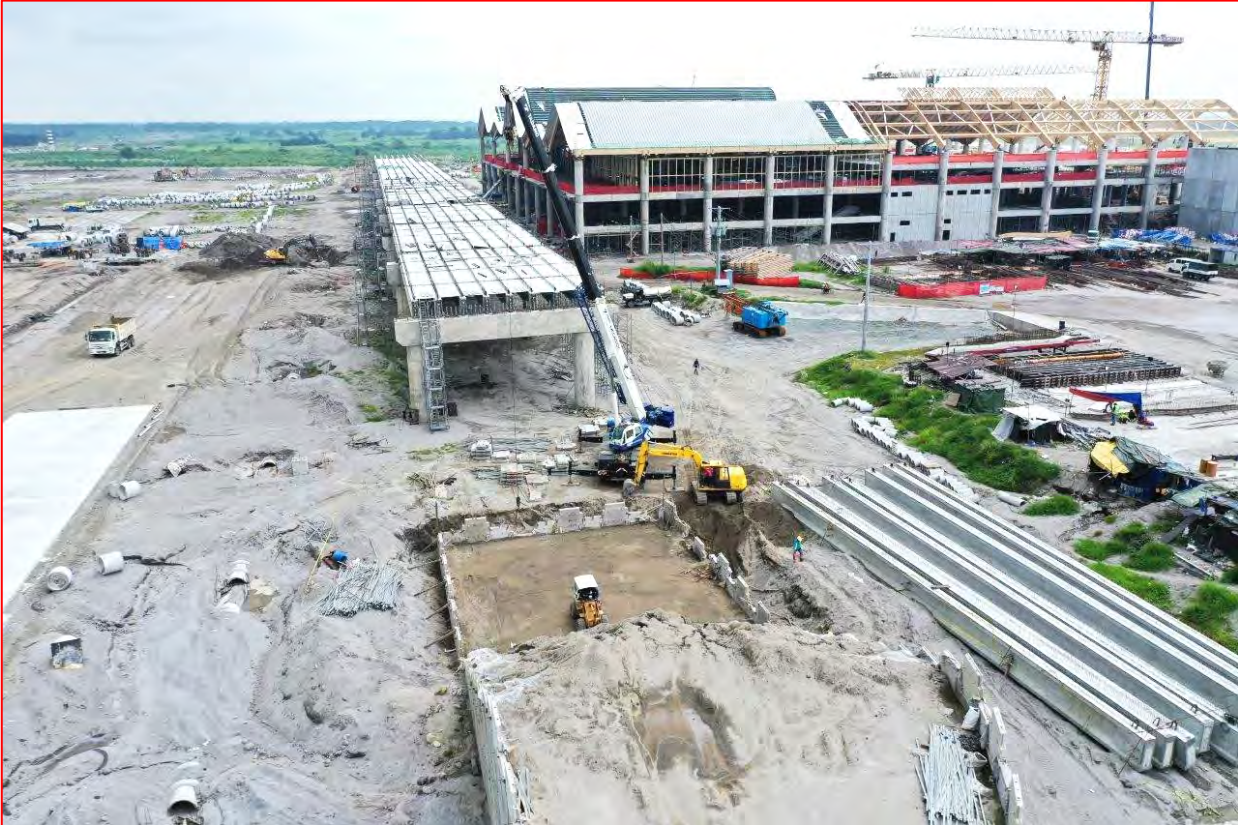
Figure 19: Abutment A – MSE Wall installation in Elevated Road.
