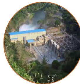
Angat Hydroelectric Power Plant (AHEPP) - Rehabilitation and O&M of Auxiliary 4 & 5 (under development)
