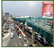
NAIA Expressway Phase (II)
